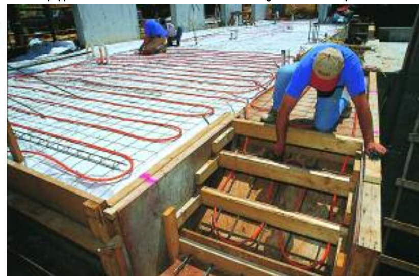
Barrier-equipped RadiantPex installs in a concrete slab. Imagine snow-free steps.
