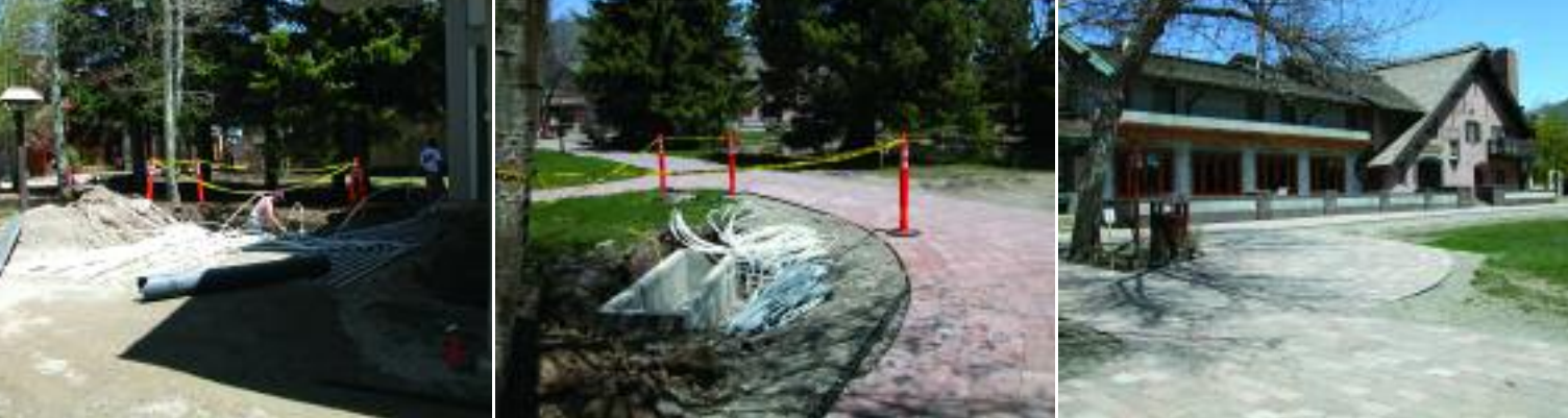
RadiantPex installs in sand below concrete pavers and will join with a manifold. Imagine warm pavers instead of shovels, blades or salt.
