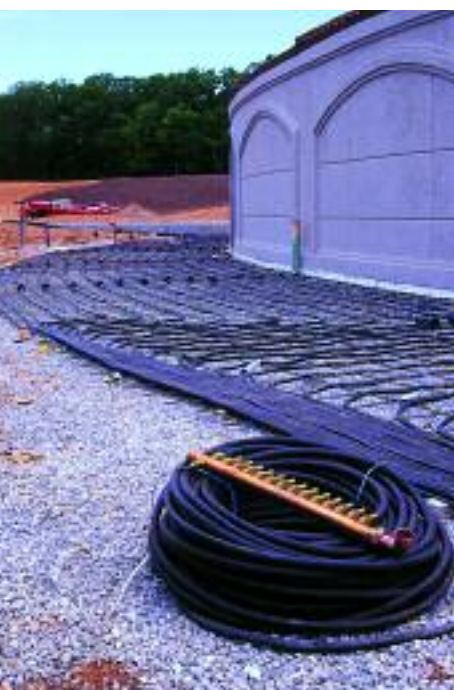
Onix tubing ready for a concrete sidewalk.
