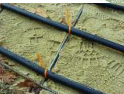
Onix tied to reinforcing wire in sand. Cover with bricks, stone, or pavers for snow-free safety.
